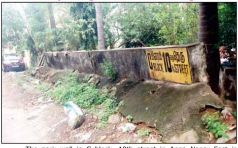
The park wall in C block, 10th street in Anna Nagar East is found in a damaged condition posing a threat to the people walking and commuting by the side. The condition is such that it could fall anytime. Proper support has to be kept to avoid the broken wall falling in the road abruptly. Entire
