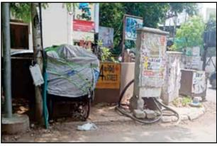
Electric cables outside the street corner of the transformer are W block 4th street in found lying loose in Anna nagar. The wires
